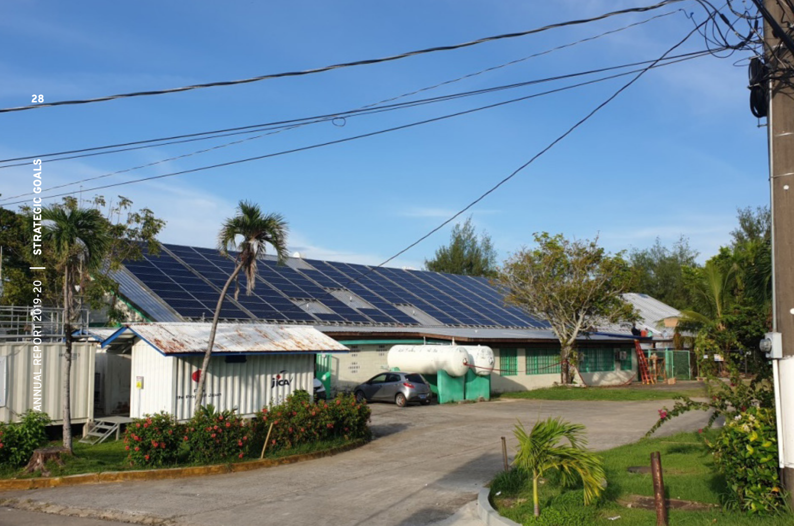
109 kW rooftop solar project constructed on the Palau Community Centre roof. Credit: MFAT.
