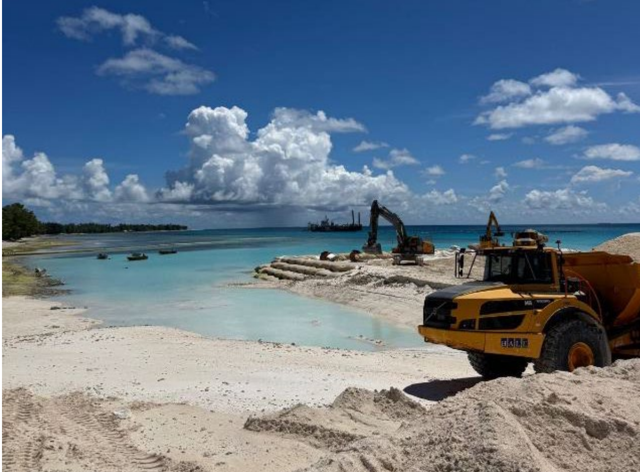
Construction of reclaimed land under the Tuvalu Coastal Adaptation Project. See p.173 for story. Credit: Rebekah Robertson, MFAT
