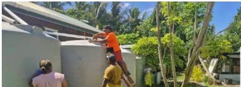
EDNRE completing installation of community rainwater harvesting system at Fakaofu, Tokelau Credit: Government of Tokelau
