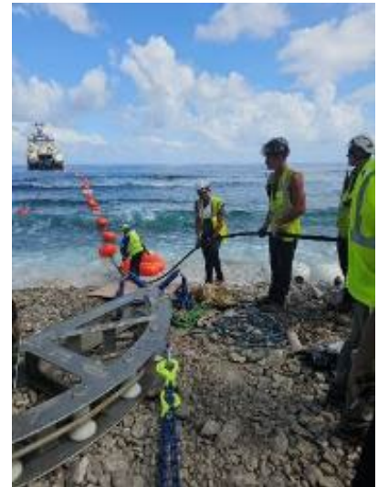
Landing of the Tuvalu Vaka Cable in Funafuti. Credit: Australian Infrastructure Financing Facility for the Pacific
