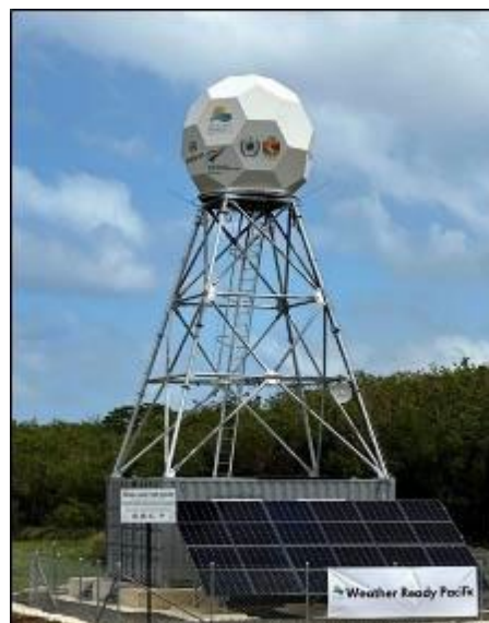
Weather radar at Fua'amotu International Airport. Credit: NZ MetService
