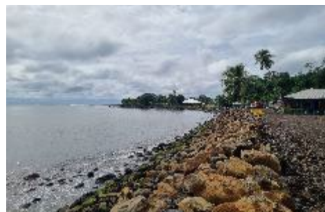
Newly constructed Lau'i'i seawall, Samoa. Credit: MNRE
