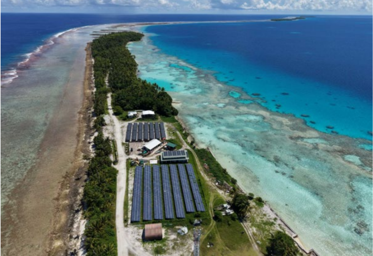
Upgraded solar energy system in Nukunonu, Tokelau. The project is renewing and expanding Tokelau's renewable energy infrastructure, improving access to reliable clean energy, and reducing Tokelau's reliance on expensive imported fossil fuels. Commissioning of the upgraded system in Nukunonu is planned by August 2026. Following completion of similar upgrades in Atafu and Fakaofu in late 2026, most Tokelau's electricity needs will be generated by solar energy. Credit: SPREP
