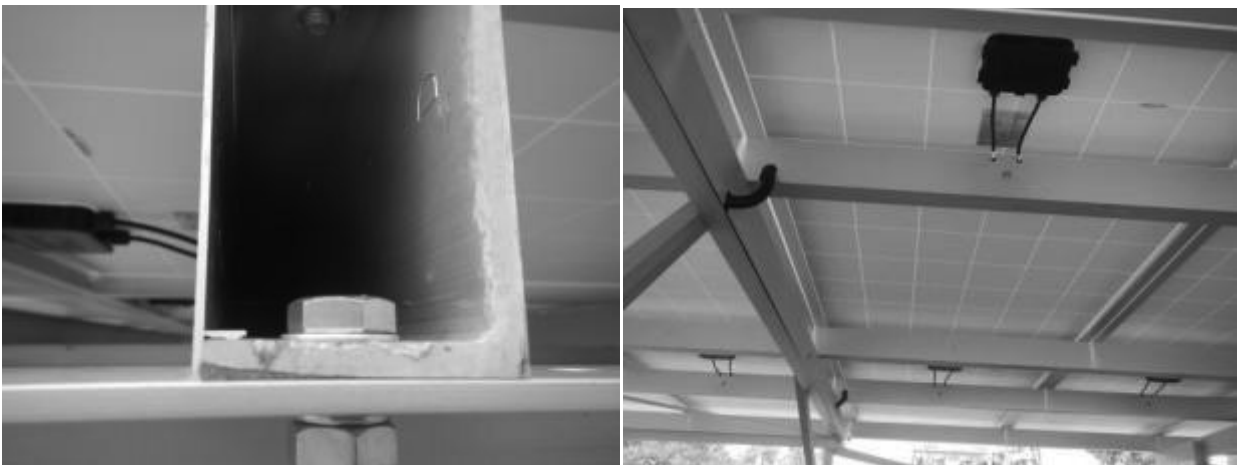
Figure 40: Array frame detail showing general framing and bolts
