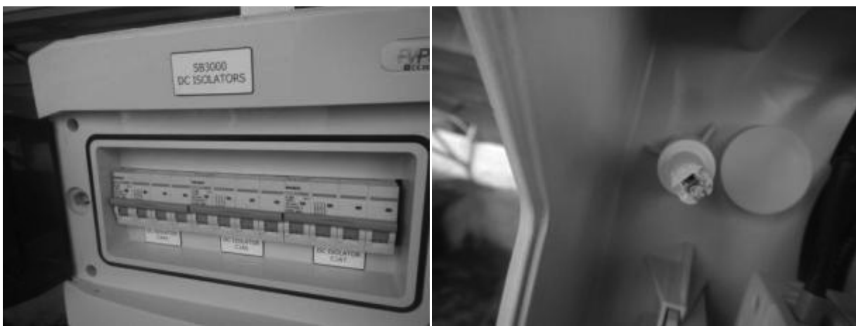
Figure 45: Isolator labelling (left) and screw mount (right)
