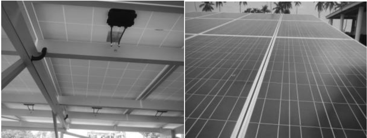
Figure 42: Typical condition of panels
