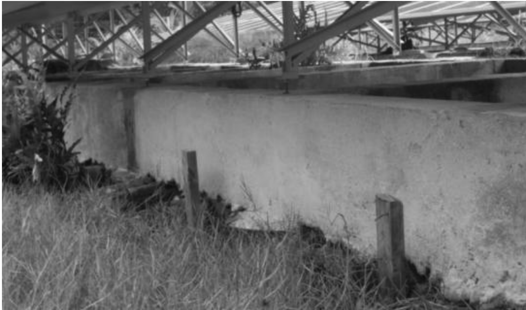
Figure 5: Foundations in swampy ground supported by wooden logs
