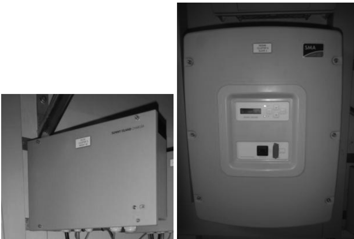
Figure 14: Charger with faulty indicator light (left) and Sunny Island missing SD card (right)
