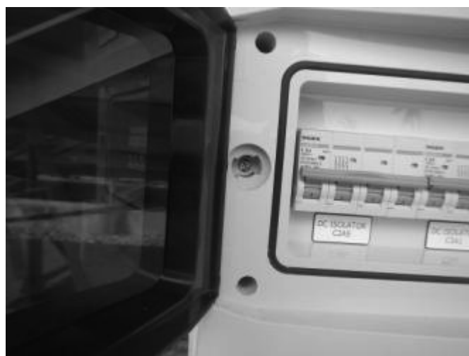
Figure 46: Isolators free from wasp nests
