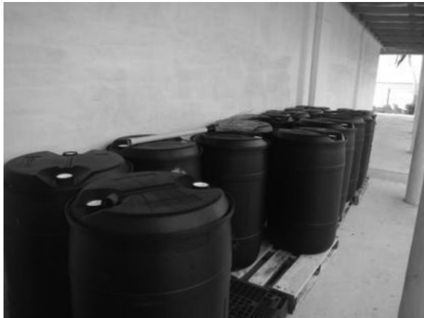
Figure 69: Spare battery acid stored under cover
