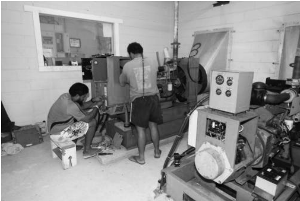
Figure 68: Generator maintenance work underway
