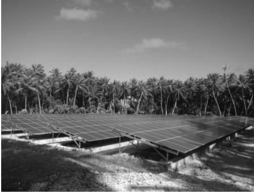
Figure 96: Minimal vegetation around panels; shading on front row from trees on adjacent land
