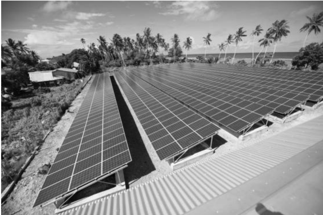
Figure 63: Area around the array is very clean and tidy
