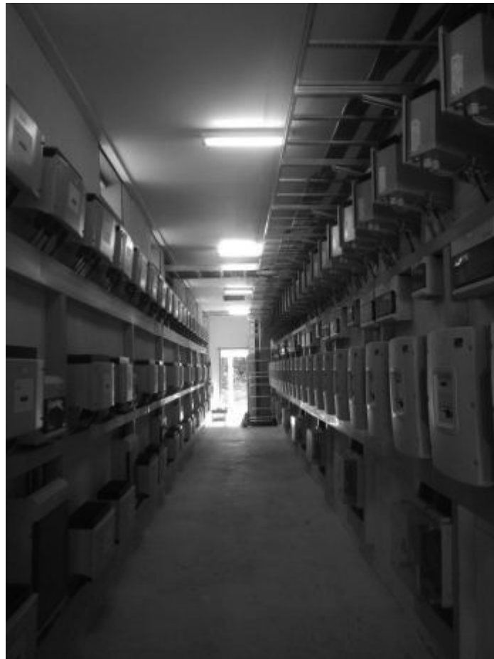
Figure 98: Inverter room
