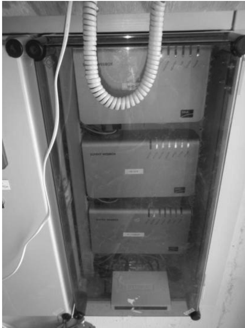
Figure 55: Webboxes have no internet connectivity (red light)
