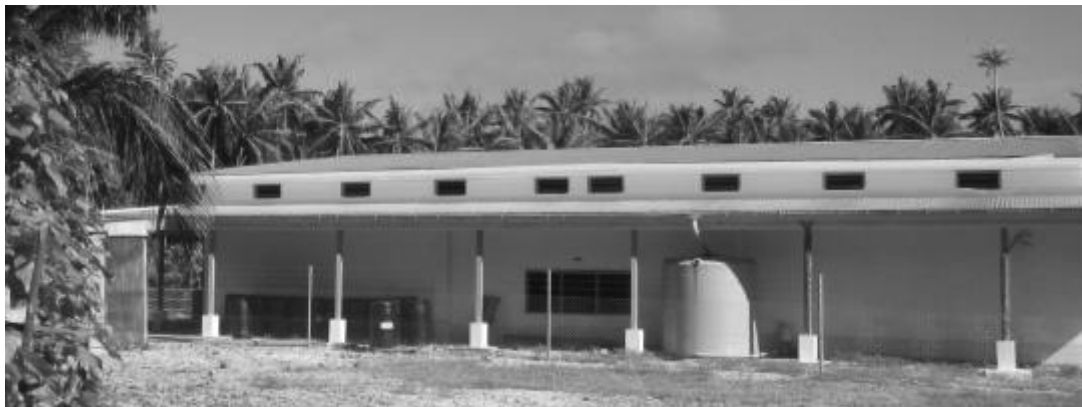
Figure 103: Battery acid drums
