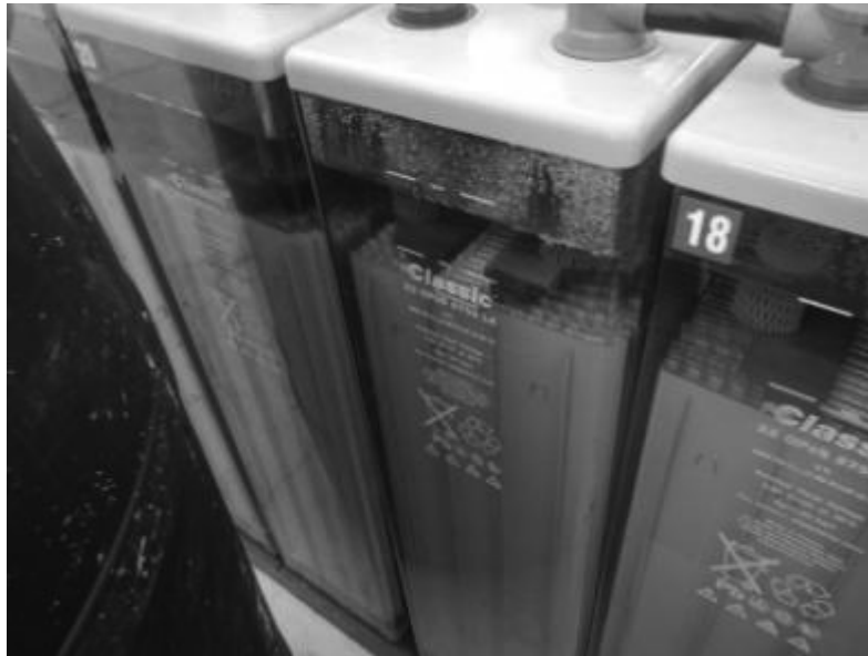
Figure 101: Battery electrolyte levels on old and new cell
