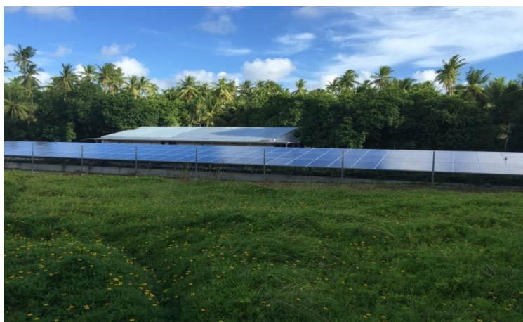
Figure 9: Solar Panels on Fakaofu
