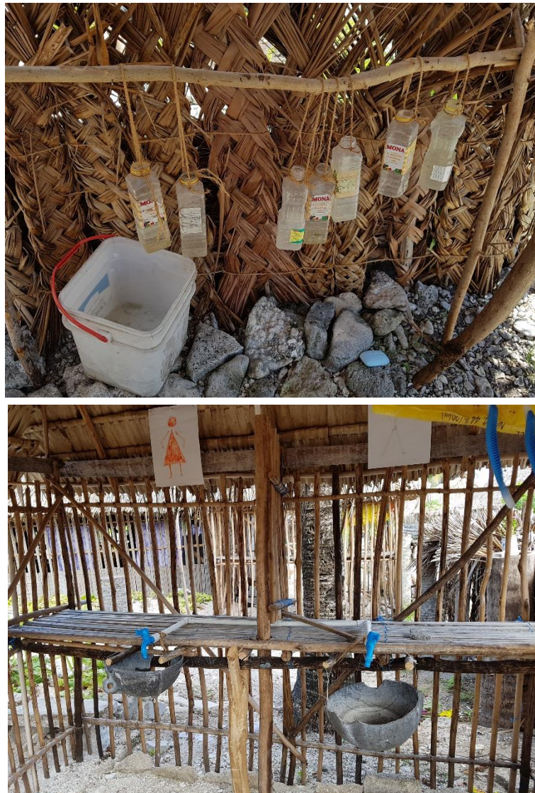
Figure 2 - Handwashing facilities installed in Ueen Abaiang JSS (top) and Sunrise PS (bottom)
