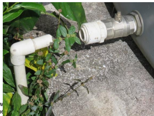
Figure 2 Vaivase Primary School broken pipe from water tank
