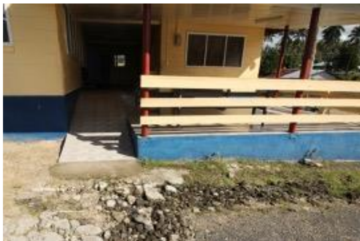
Photo 2: Damage to access ramps at Saanapu health centre, June 2018
