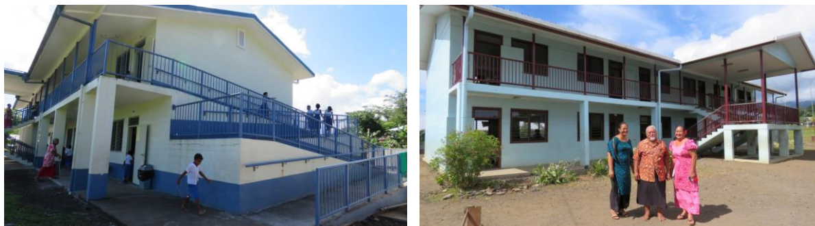
Figure 1 Standard design for ramp to classroom and Vaivase Primary School – lack of access between classrooms
