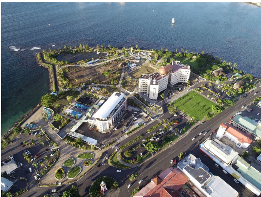
Figure 3. Post-development of the Events Space and Clock Tower Boulevard
