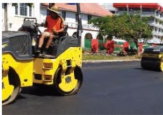
Sealing works of the Event Space 2 in progress
