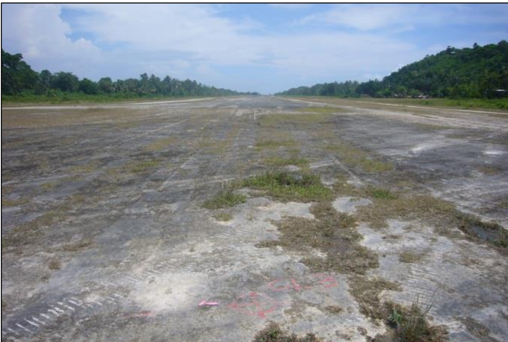
Figure 5 – Munda Airstrip Prior to Upgrade Works
