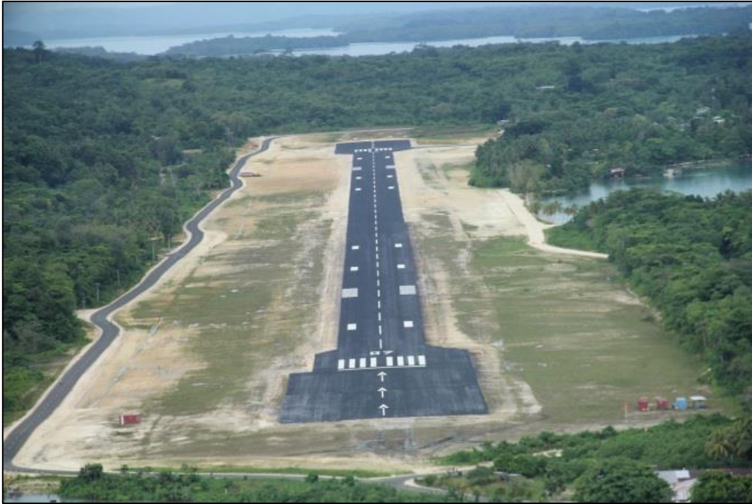
Figure 6 – Munda Airstrip following Phase 1 Upgrade Works
