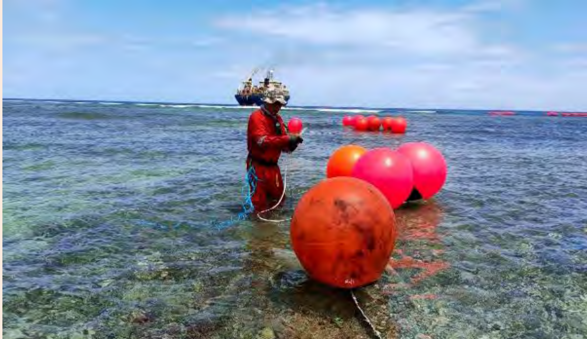
Landing Tokelau's first international subsea cable onto Atafu, Tokelau's northernmost atoll. The international cable went live in September 2023 across all three atolls, with services operated by Teletok, Tokelau's telecommunications provider. Tokelauan communities now have significantly improved international and inter-atoll internet connectivity at a lower cost, and with greater availability and reliability. Credit: McCann Consulting Ltd, 2022
