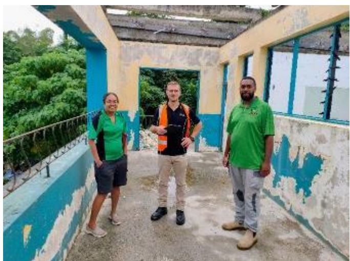
Engineering assessment of a school in Port Vila. Credit: © CHartnett
