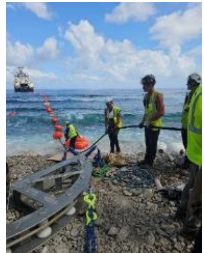
Landing of the Tuvalu Vaka Cable in Funafuti. Credit: Australian Infrastructure Financing Facility for the Pacific
