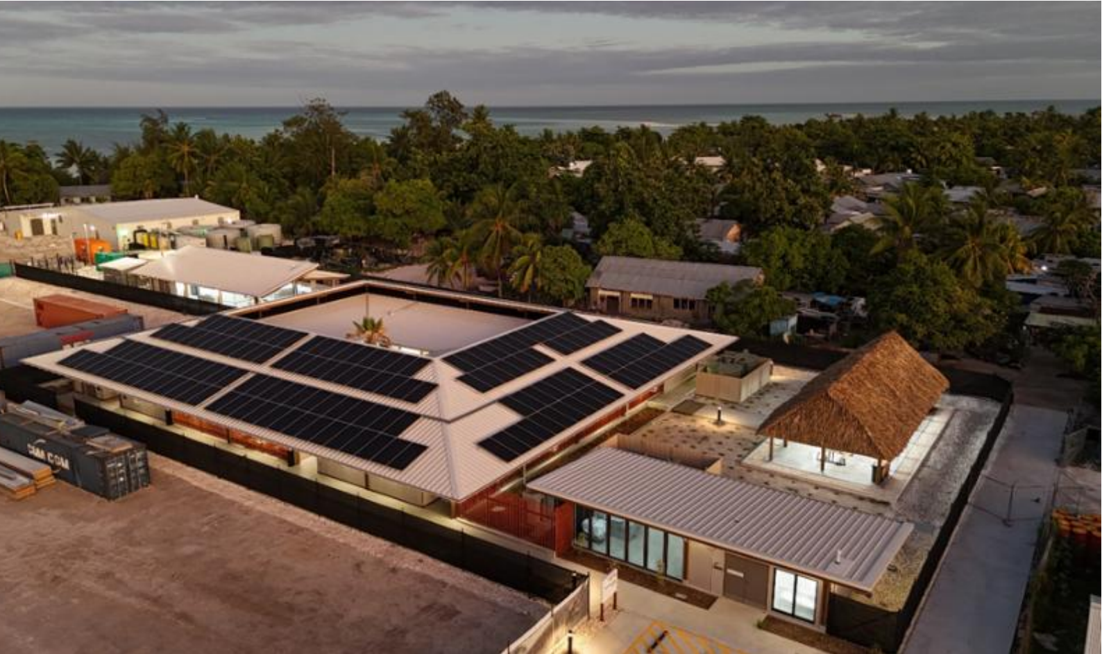
Aerial view of the New Betio Hospital site in Kiribati, showing the maternity ward, paediatric ward, kitchen, laundry, staff areas and traditional maneaba funded by New Zealand and constructed by Reeves International, with engineering services provided by Egis. Credit: Reeves International
