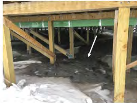
Visible ACM fragments under the Administration building
