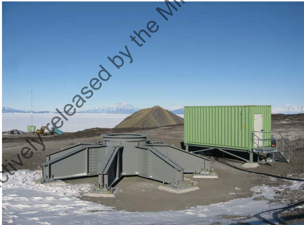
Figure 54: Steel spider framework bolted to the concrete foundation blocks.
